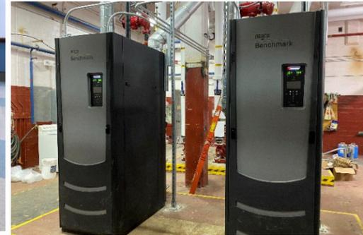
New Hot Water Condensing Boilers
